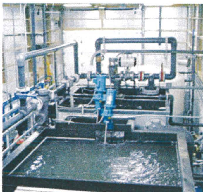
Inclined Plate Clarifier
